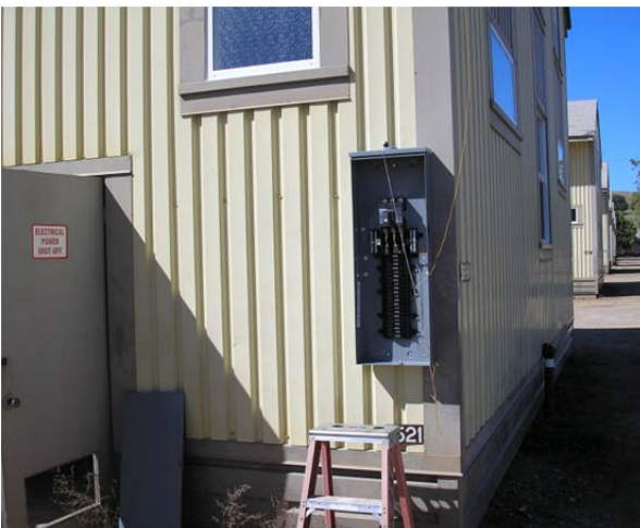
Installing the new subpanel
