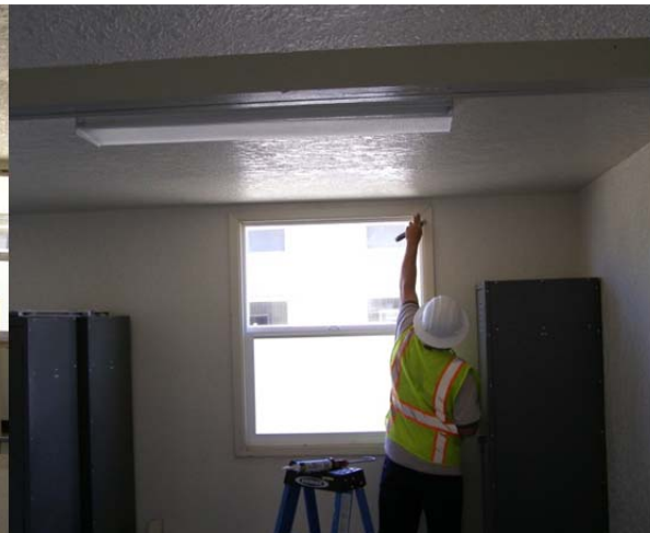
Caulking the new trim
