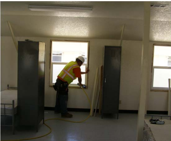
Trimming the new windows
