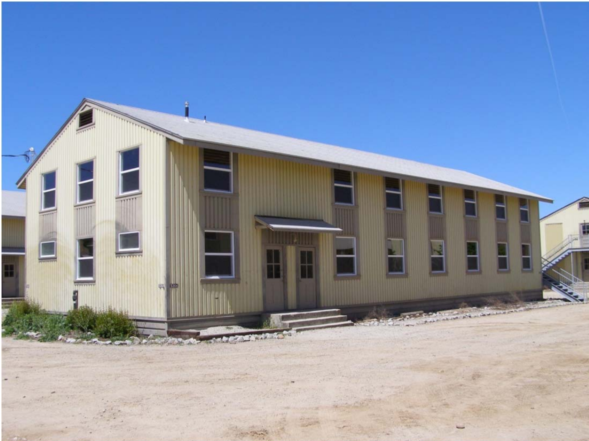
This work on the above building is complete.
