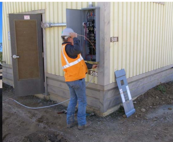
Connecting the ground wire to the subpanel.
